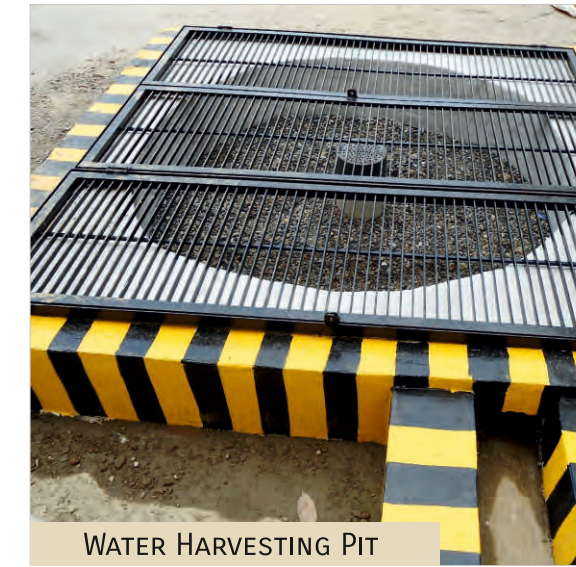
WATER HARVESTING PIT
